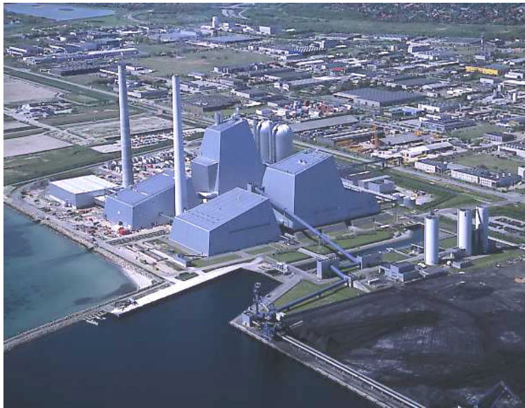
Figure 6: Avedore 2 Bioenergy Power Plant (taller unit)
