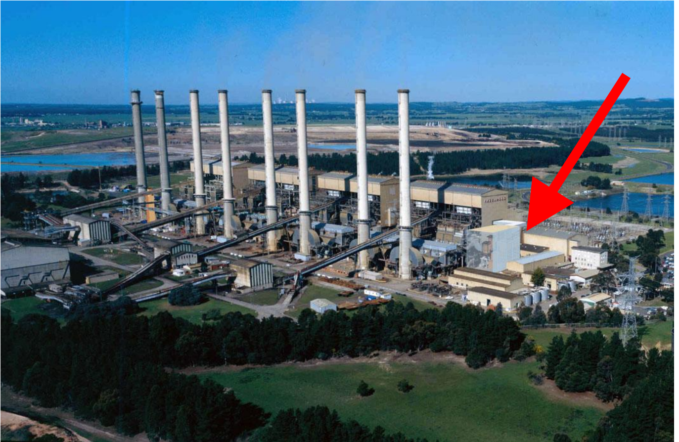
Hazelwood Power Station with Artists Impression of Demonstration Coal Drying Plant
