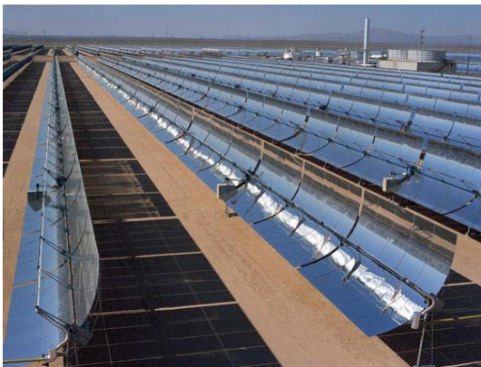
Parabolic troughs at Kramer Junction, California (Credit: Warren Gretz (DOE/NREL Photographic Information Exchange))
