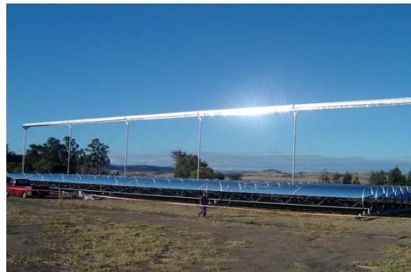
Linear Fresnel pilot plant at Liddell Power Station, NSW Australia. (Credit: Solar Heat and Power)
