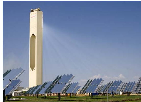
PS10 Power Tower ( Planta Solar 10) – near Seville in Spain (Credit: Solucar)
